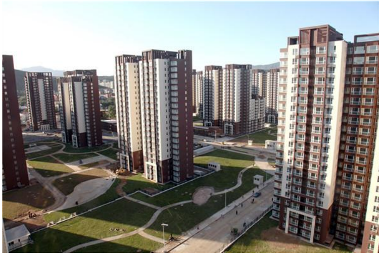
Photo: Beijing Urban Construction Group
